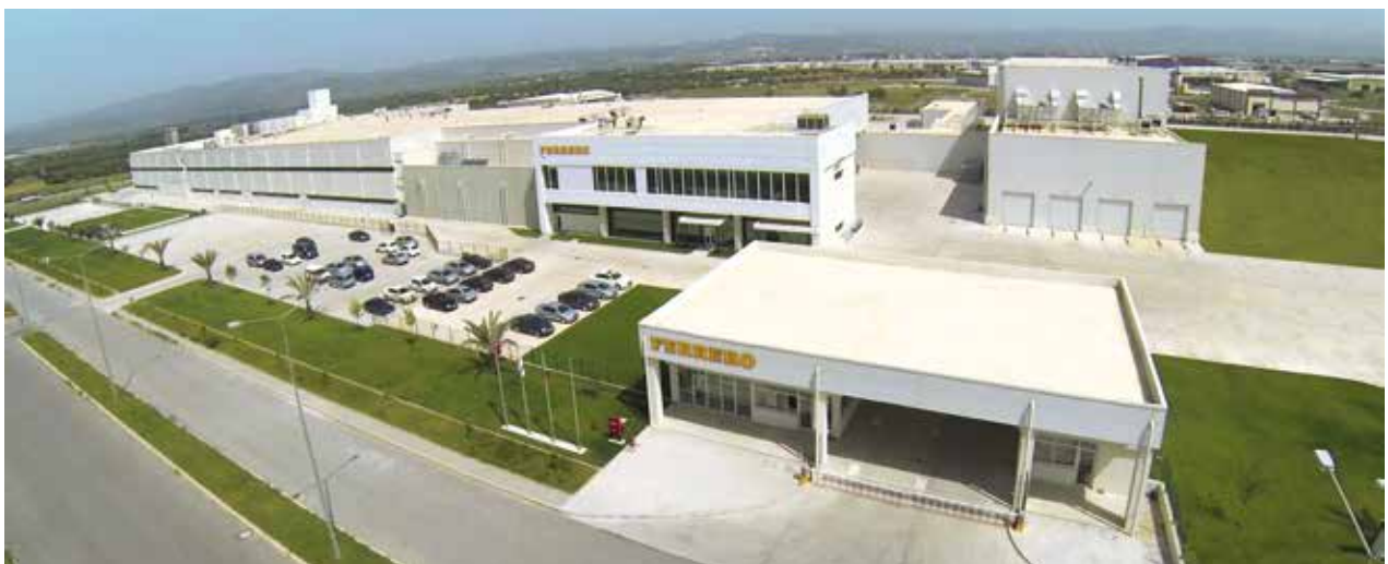
New Ferrero production plant in Turkey
